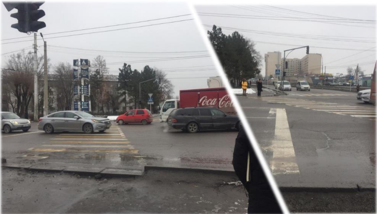
Figure 3: Crossroad of Maldybaev – Akhunbaev location before upgrades
